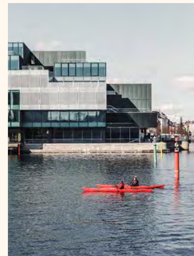
BLOX is a natural part of the harbour's transformation from industrial infrastructure to recreational blue park.
