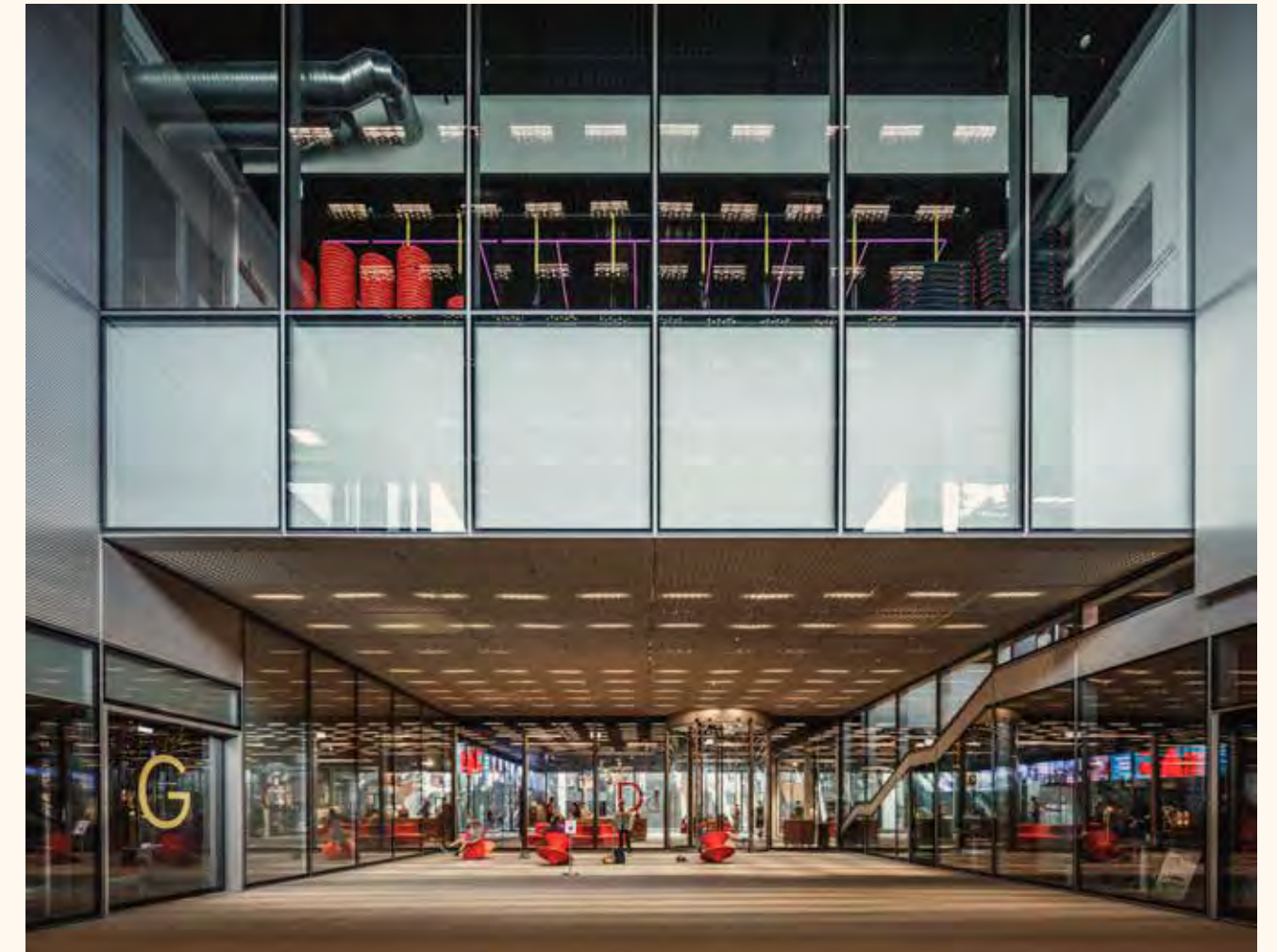
DAC Passage. The underpass is located two storeys below ground. It is a public space with access to the harbour front and entrance to the Danish Architecture Center.
