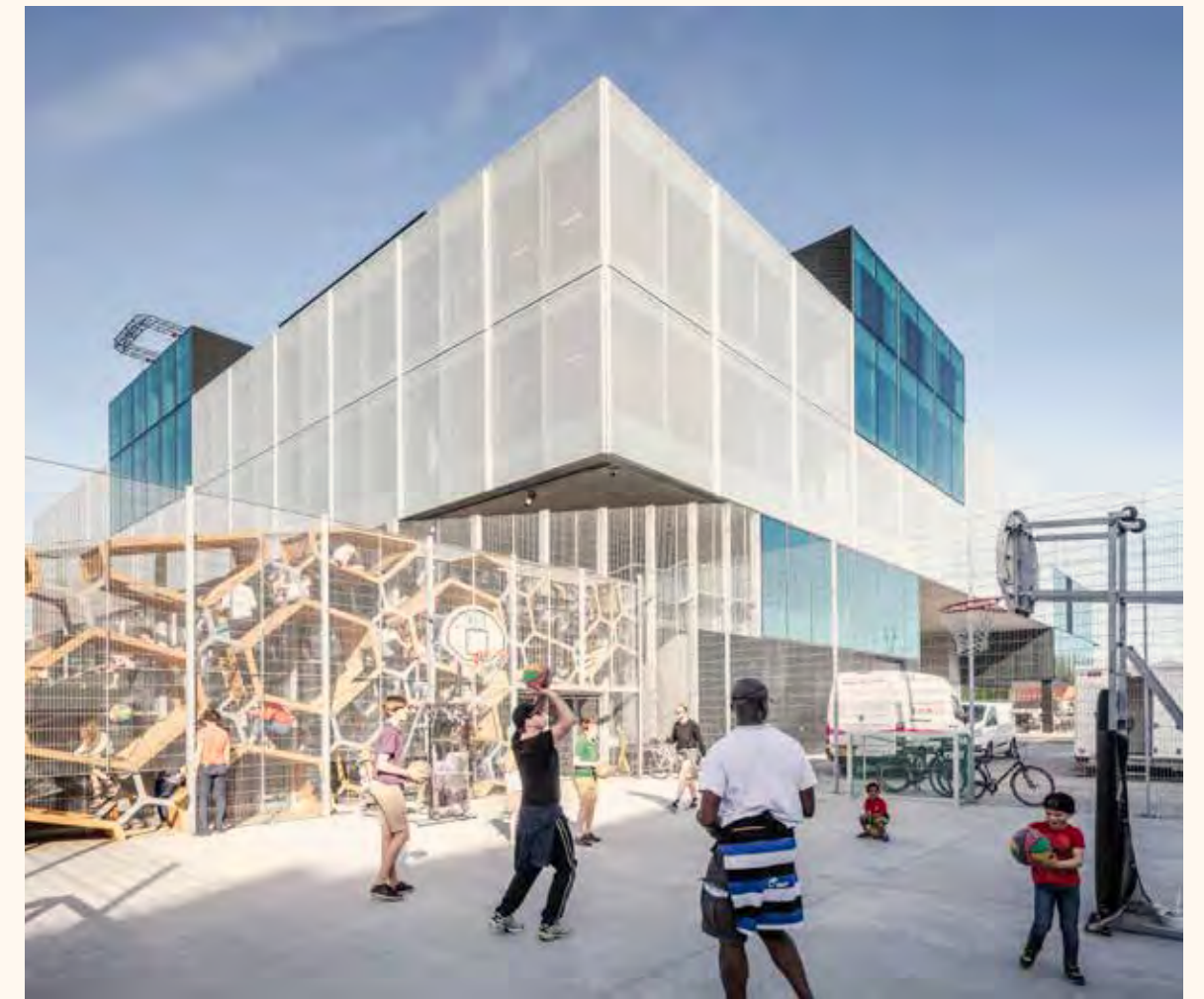
The public playground by BLOX with a ball cage and a climbing rack, seen from Vester Voldgade. Behind the climbing rack there are other playground facilities.
