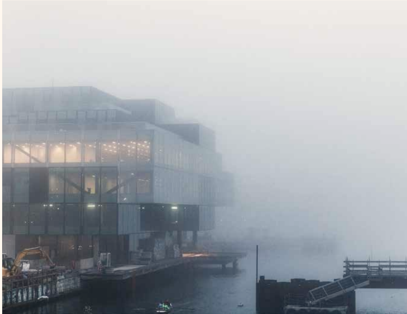
BLOX under construction. Like a Venetian palazzo, the building sits directly on the water. 2017.
