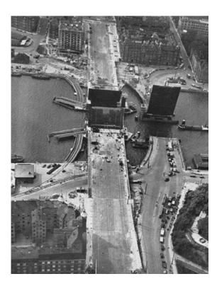
The current Langebro with two bascules was built next to its predecessor during the early 1950s. Note that the railway was located south of the current bridge on a low swing bridge.
